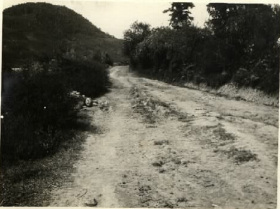
Rehab Djalan Alur Ines.
