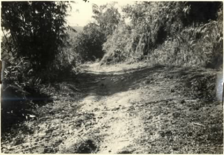
Rehab Djalan Burui Pepalang.
