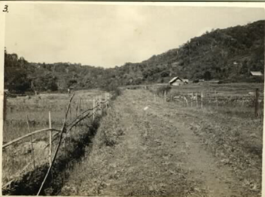
Rehab Djalan Pipalang.
